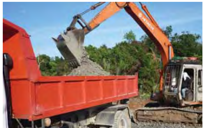
Loading of crusher runs for grading and compacting estate road.
