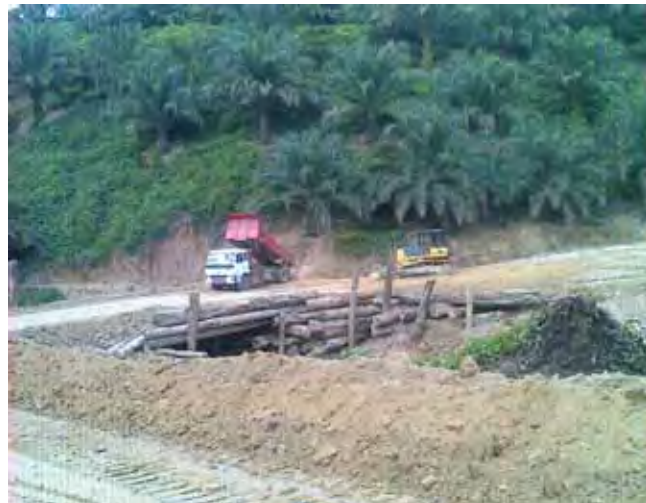
Repair of bridge in Millian-Labau Plantations, Sabah
