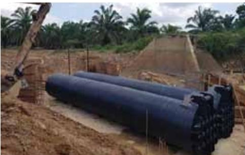
*High Density Polyethylene (HDPE) culvert installation in Batu Anam Estate*
